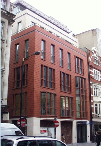
Hanover Street, London Curtainwalling and Sliding Doors
