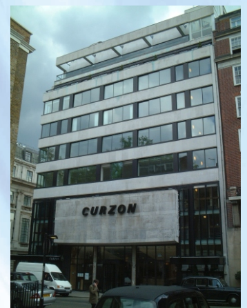
Curzon Street, London New Curtainwall and Sliding Windows to Grade 1 Listed Building
