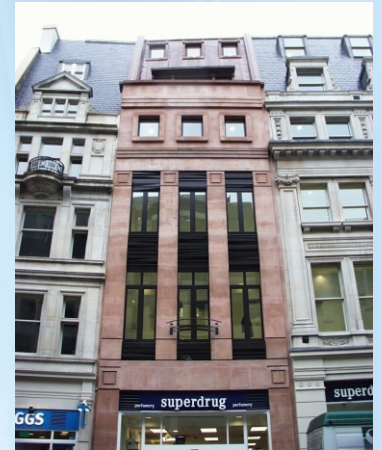
Eastcheap, London Curtainwall, Windows and Doors
