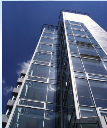
Fountain House, Reading Staircase Curtainwall and Smoke Vents
