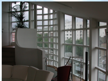
Elystan Place, London Faceted Curtainwall to Tower
