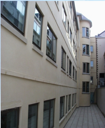
Esplanade, Jersey Curtainwall, Windows and Doors
