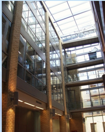
Aviation House, London Fire Rated Curtainwall and Doors
