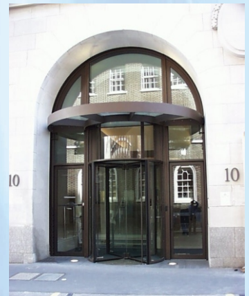
Old Jewry, London Entrance Screen with Revolving Door, Pass Doors and Canopy
