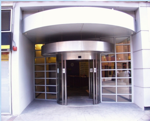
Fountain House, Reading Complete Entrance and Canopy
