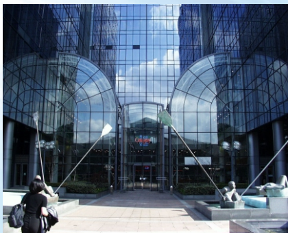
Harbour Exchange, London Structurally Glazed Entrance Screens and Automatic Doors
