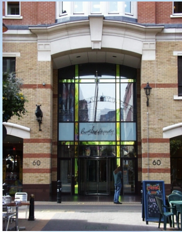
Regents St, London Entrance Screen and Revolving Door
