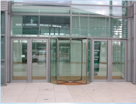
Aviator Park, Weybridge Manual Pass Doors
