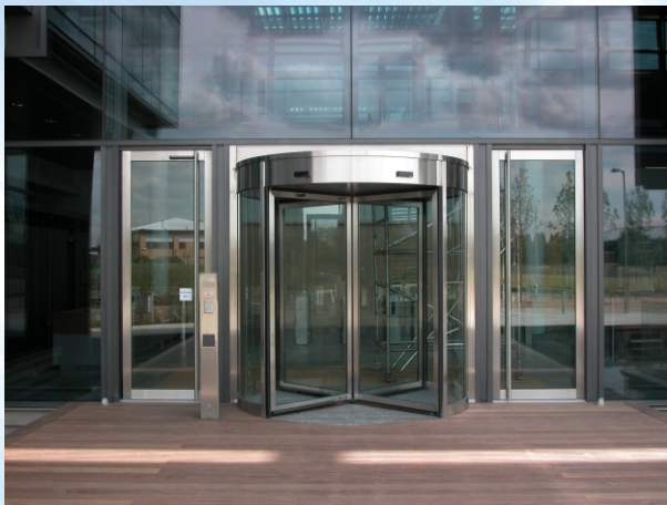
Sophus, Abingdon Disabled Access Door Adjacent to Revolving Door
