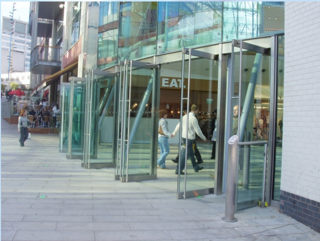
Bull Ring Shopping Centre, Birmingham Automatic Entrance Doors within Planar Screen
