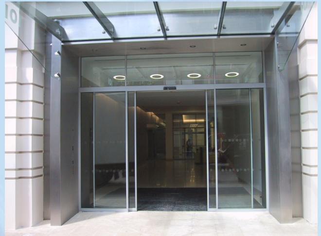
101 St Martins Lane Automatic Sliding Doors
